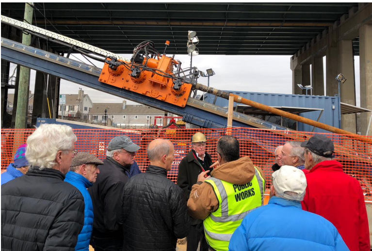
Y's Men at Sewer Drilling Project
